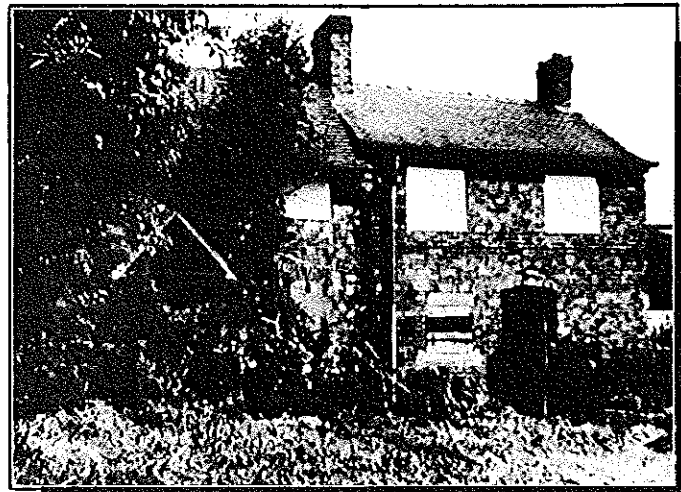
Hagg's Farm in present condition.
